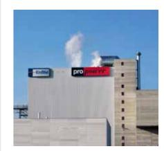
The multi-fuel combined heat and power station burns residue substances from paper production as well as recovered fuels from waste but it can also use sewage and fossil fuels as energy sources.
